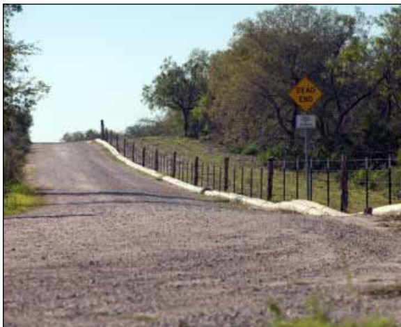
Pipes carrying water for fracking operations line a gravel road in rural Karnes County.
