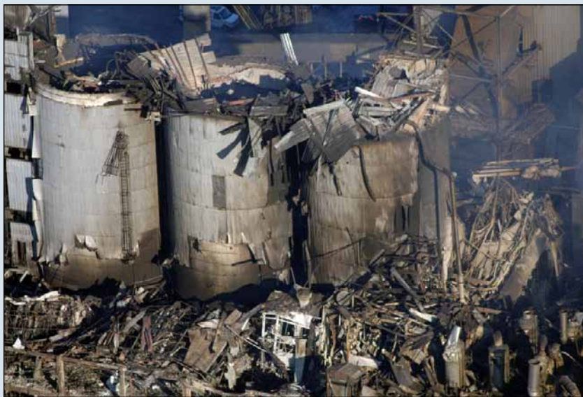
A sugar dust explosion in 2008 leveled much of the Imperial Sugar packing facility, killing 14 workers and injuring dozens more. AP Photo
