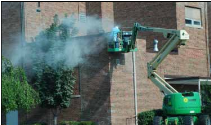
An unprotected restoration worker generates a cloud of silica dust while cutting masonry on a school in Michigan. Tom Ward
