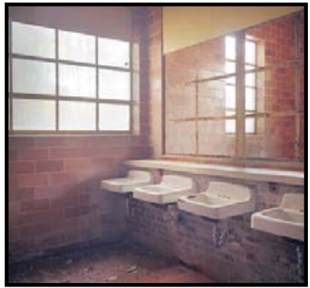
A bathroom in an abandoned school cottage.
